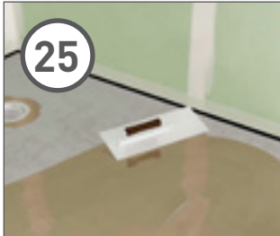
25 With a metal trowel, spread the adhesive onto the floor and coving, use a smaller spatula to apply adhesive round the drain hole.
