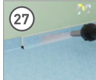
27 A heat gun can be used to warm and soften the vinyl.
