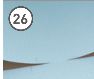
26 Ensure any dust or foreign particles are removed from the underside of the WetFlor® prior to bonding. Carefully place the sheet in position, lining it up using the check marks.
